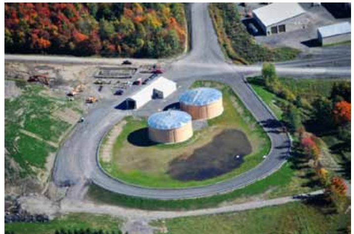
TOP: Construction of new scale foundations and the building addition at the DANC SWMF
